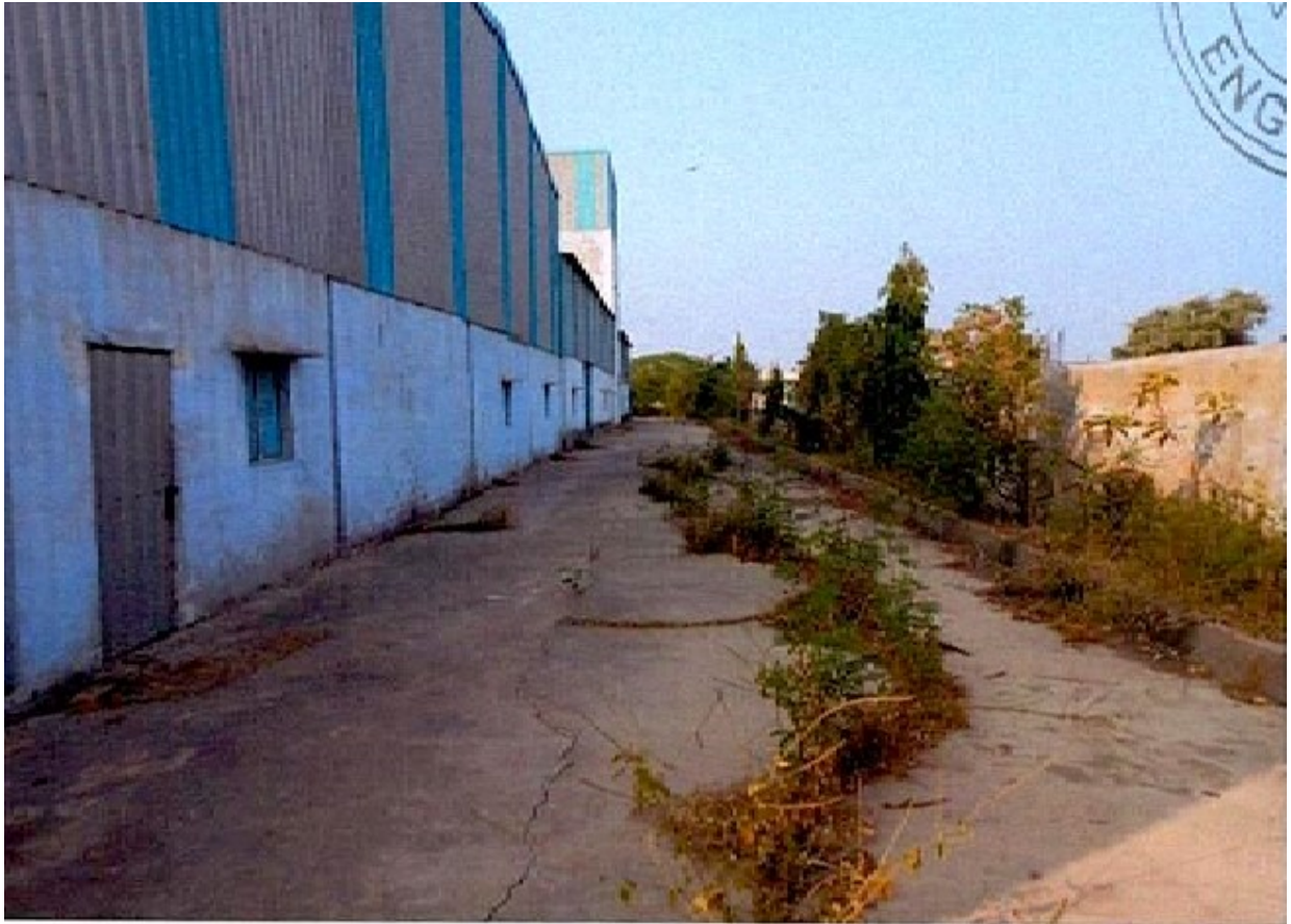
Photographs of Factory Land & Building page no. 8-11
